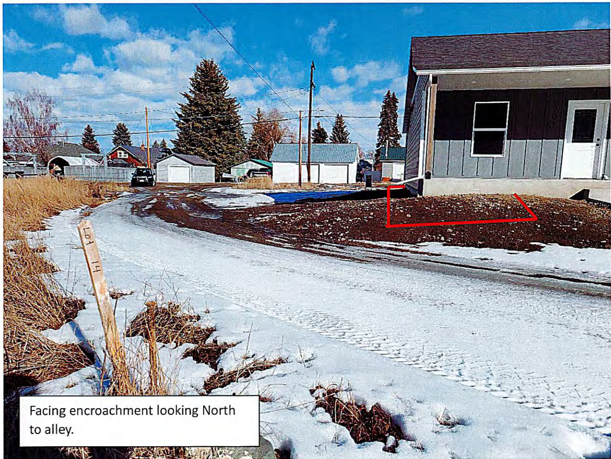
Facing encroachment looking North to alley.
