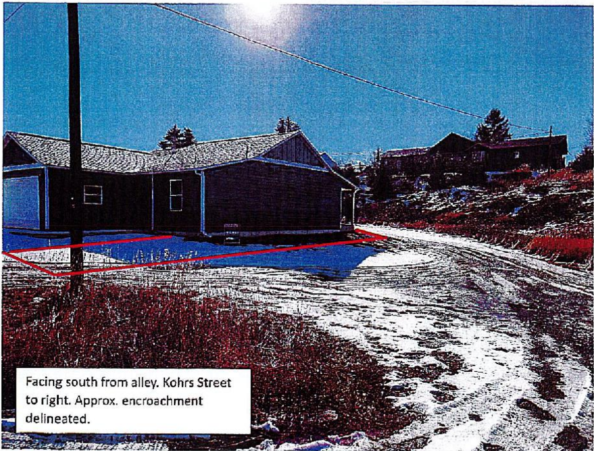
Facing south looking towards Montana Ave. Kohrs Street on right. Approximate encroachment delineated.
